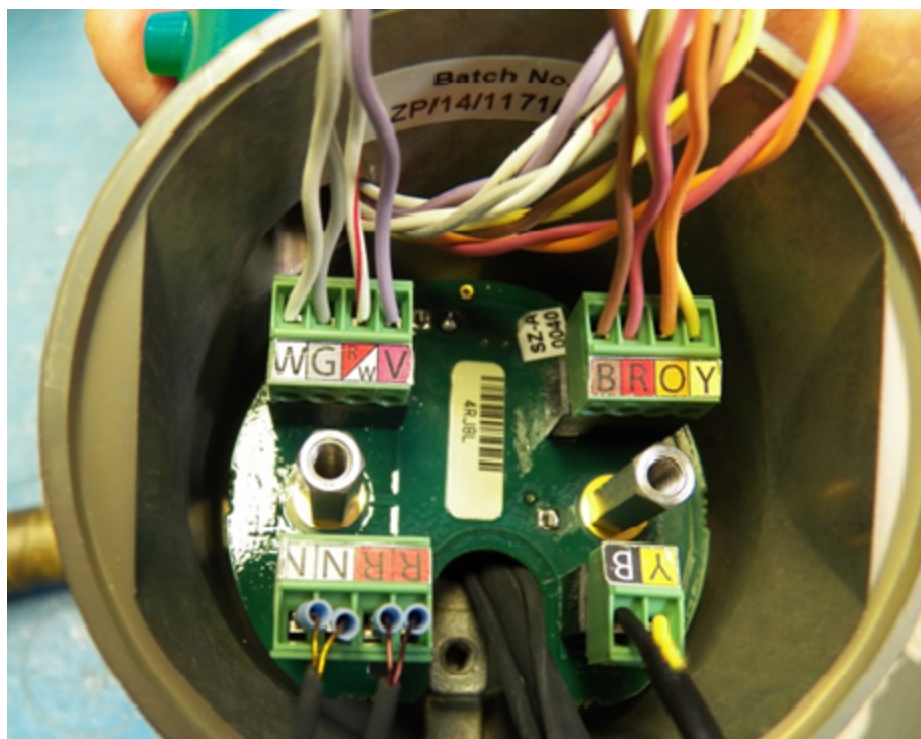
Figure 5 - Terminal Blocks in the Junction Box
